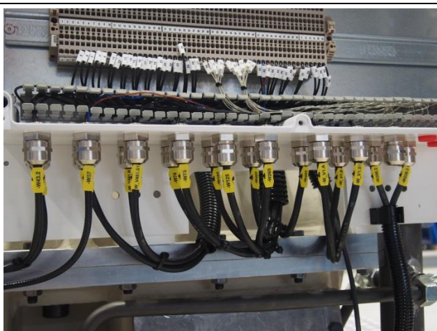
Figure 9 Connections on the terminal box
