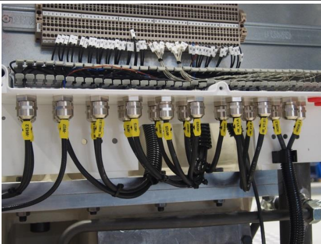
Figure 9 Connections on the terminal box
